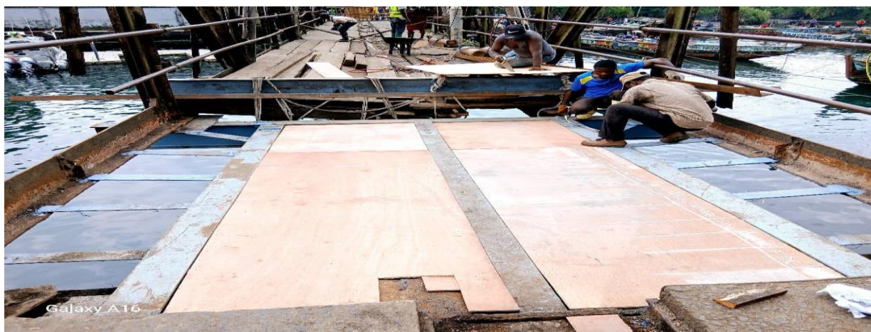
Bibunde Bridge Idenau – repaired by CDC to support operations while improving community access (CSR)
